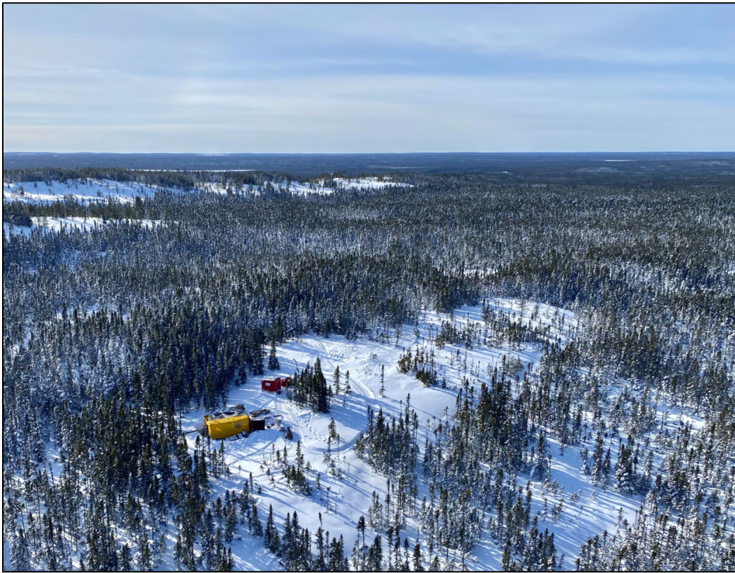
Figure 2. Drill Rig at Cisco Project
